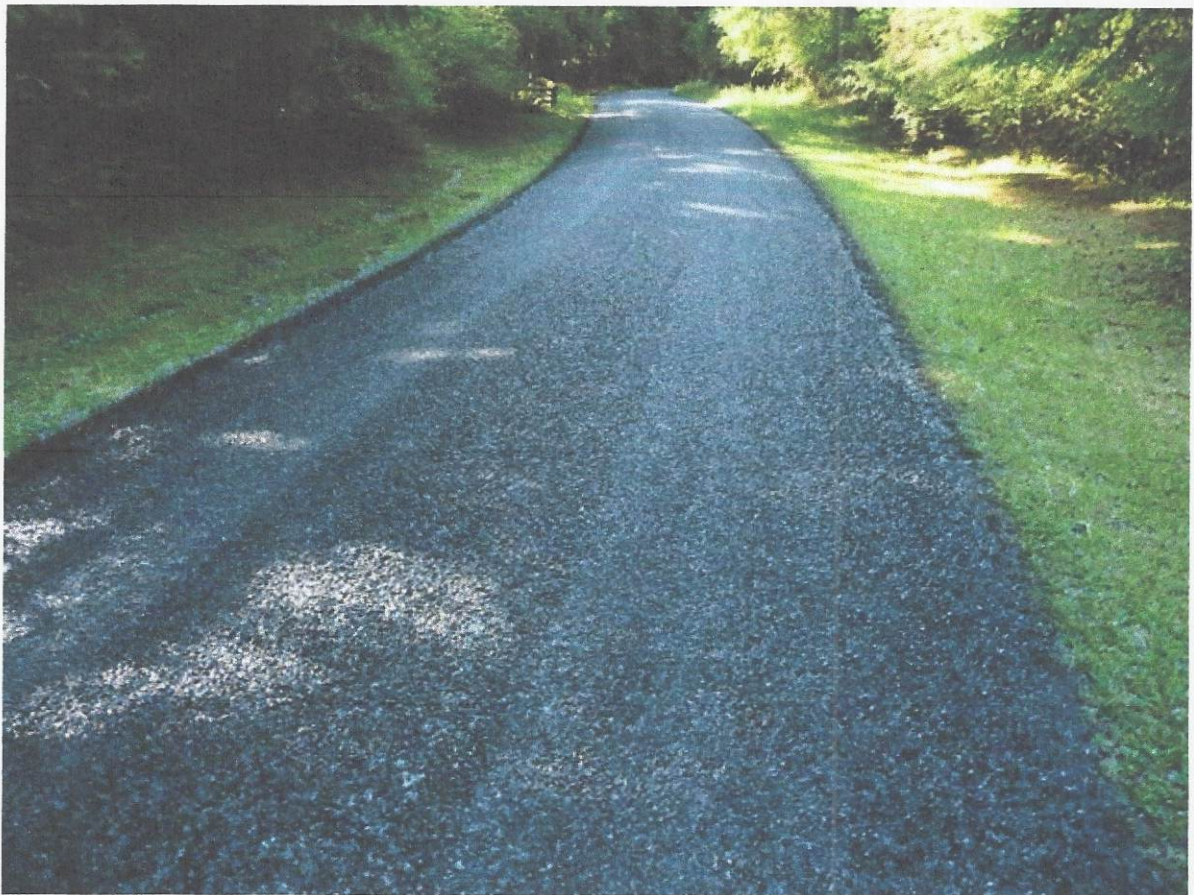
Finished road after fog seal.
