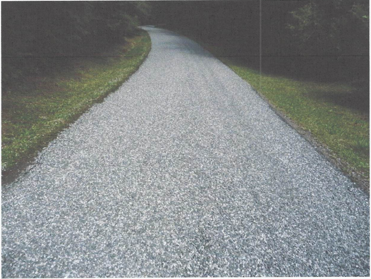
Road after chip sealing.
