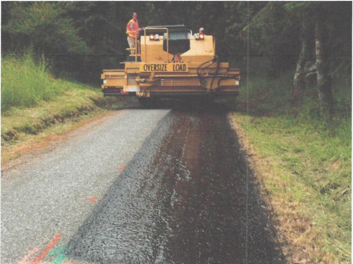
Applying gravel to a patch area below Rockledge road
